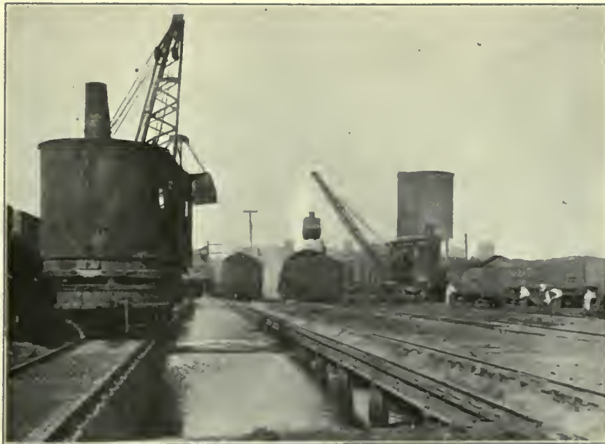
FIG. 652. FACILITIES TO BE ABANDONED. Locomotive ash-pit of the Chicago & Western Indiana Railroad at 49th and Butler streets. This double pit is equivalent to a single pit 450 feet long. It accommodates more than 100 locomotives daily. In the event of electrification, this structure will be rendered worthless in its present location. Approximately 5 per cent of its original cost of $30,000 could be recovered in salvage.
